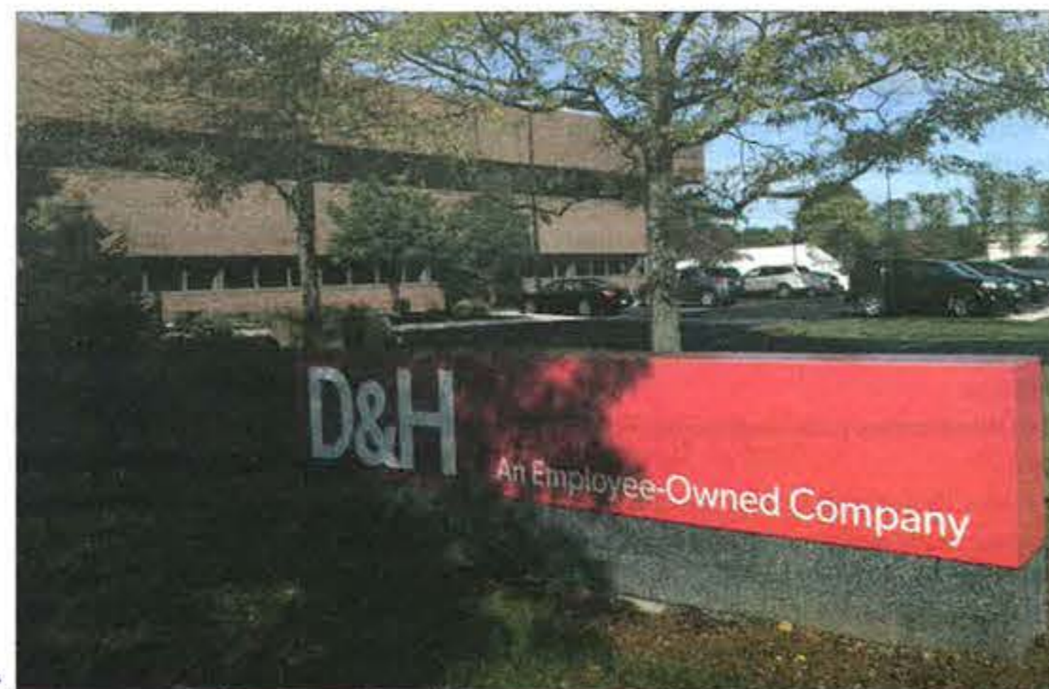
D&H Distributing, an employee-owned company and one of the largest privately-held companies in the country, recently completed its move to its new home in the former Amp Inc. and Tyco Electronics headquarters in Lower Paxton Township.
